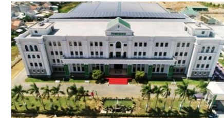
Pymepharco II in Vietnam Capacity expansion for Solids built for future growth
